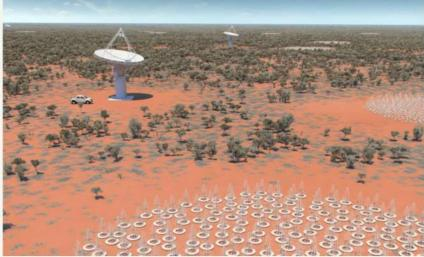
Radio Telescopes: These detect radio waves from space. The SKA is a new radio telescope project, currently in the design study phase, which will have sensitivity 100 times greater than the most sensitive radio telescopes of the present generation, and an ability to survey the sky up to 1 million times faster.
